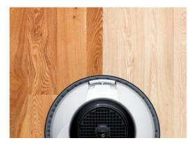
Overlap the previous sanding track by approximately half to ensure that, if present, all previous coatings are removed and that a smooth even finish is obtained.
